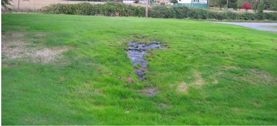
The above photo shows a leaking septic mound in the BC interior: the mound system is used where conventional septic fields cannot be built due to impermeability (or excessive permeability) of the soil. Septic liquid waste is supposed to be filtered by mound sands but if the soil permeability is too low, liquid is not absorbed fast enough, resulting in surface ponding of unsanitary liquids.
